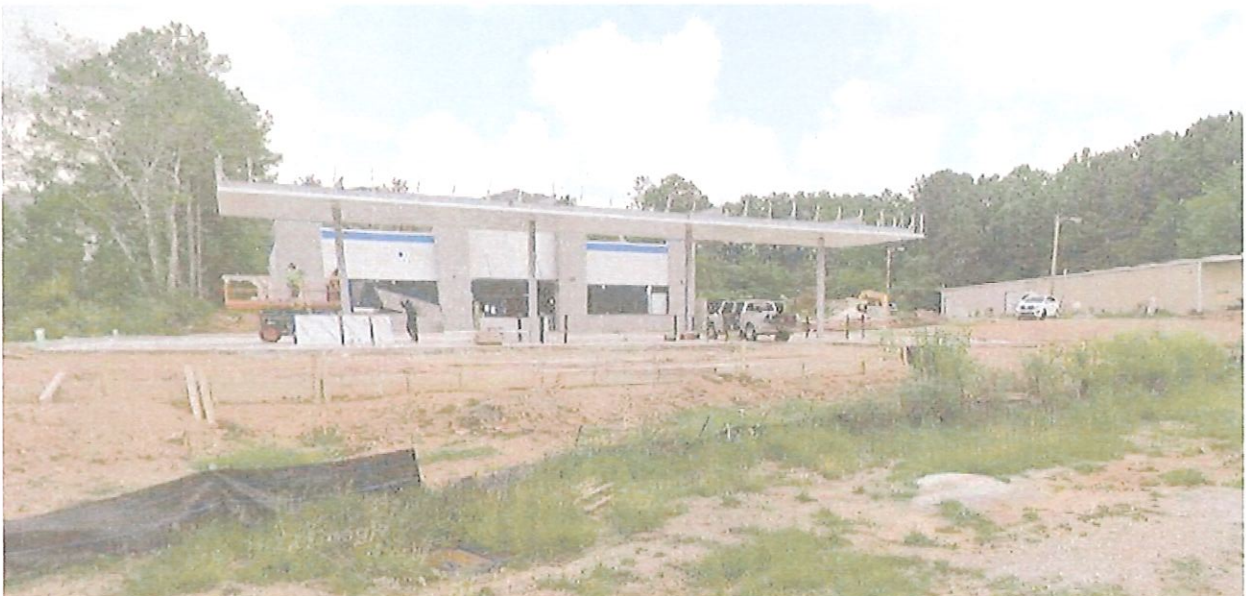
Figure 2: AAA22-000002 6030 Hillandale Drive
