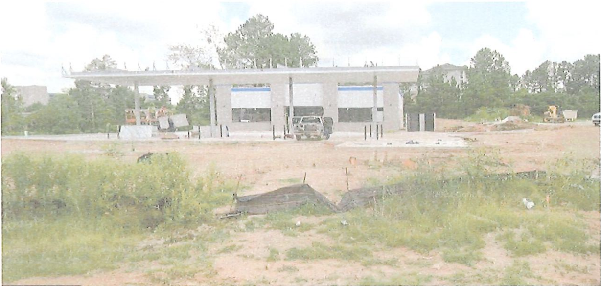
Figure 1: AAA22-000002 6030 Hillandale Drive
